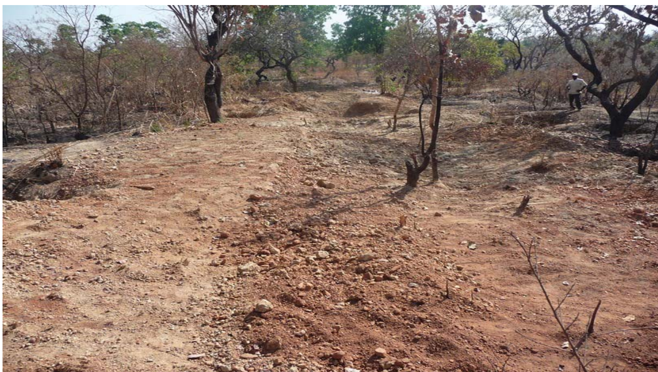
Backfilled trench at Bulenga Prospect
