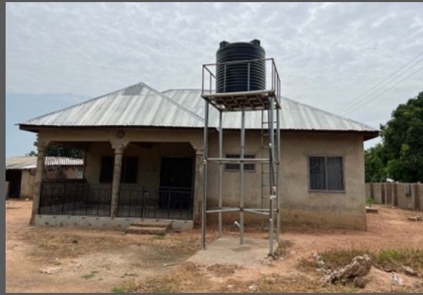
Castle installed bore hole, pump and storage tank at Sombo village
